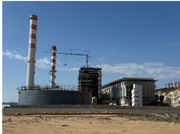
Figure 33: Porto Empedocle desalination plant exterior. Photograph taken by author, March 11, 2026.
