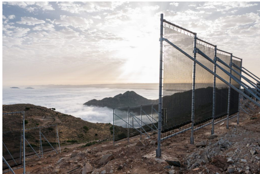
Figure 38: Fog-harvesting “CloudFisher” nets installed on Mount Boutmezguida in the Anti-Atlas Mountains, Morocco. Source: WasserStiftung, “Morocco: Mount Boutmezguida,” www.wasserstiftung.de/en/projects/morocco-mount-boutmezguida .
