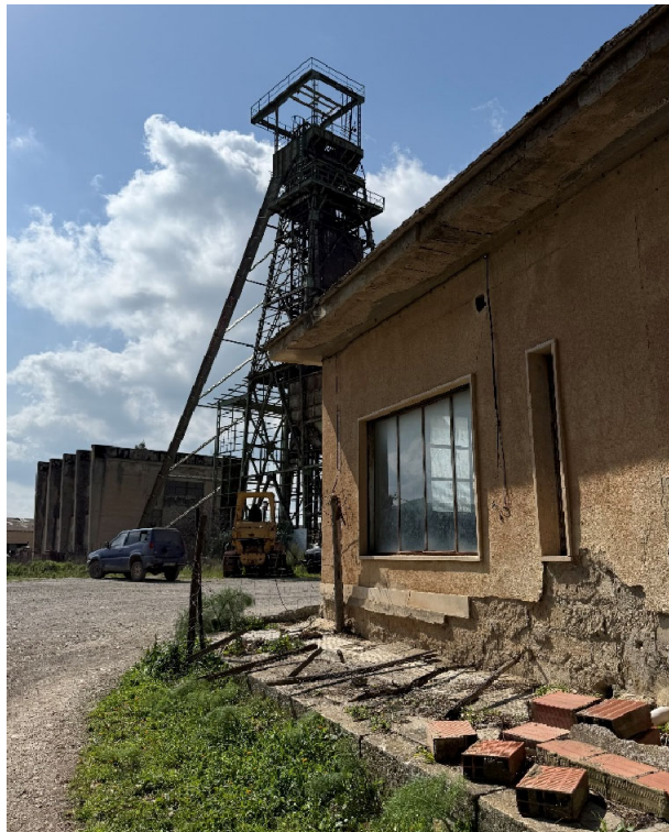
Figure 31: View of pithead tower showing material conditions of ceramic and limestone masonry. Photograph by author, March 9, 2026.
