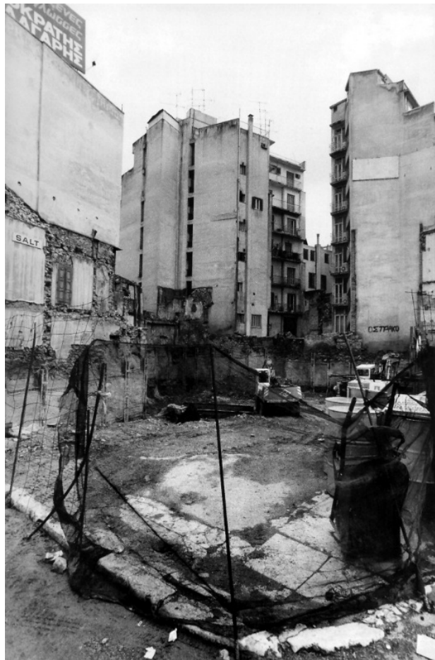
Figure 02: Construction Site . Photograph by Manolis Baboussis, 1985 -1996. M. Baboussis personal archive.
