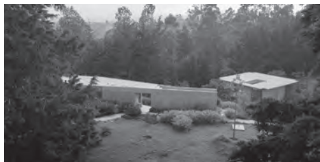
Ballen House | © LCLA OFFICE
