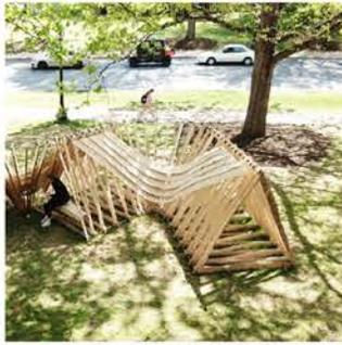
"**Easily deployed** and assembled, UNLOG unfolds several logs into an undulating and lightweight biomaterials A-frame structure... UNLOG utilizes robotic kerfing techniques and Mixed Reality tools to transform dying Ash trees into a **materially efficient, valuable resource.**"
