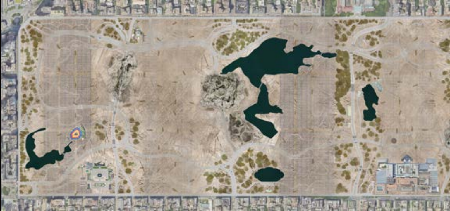
During Waste Blocks Construction Process
