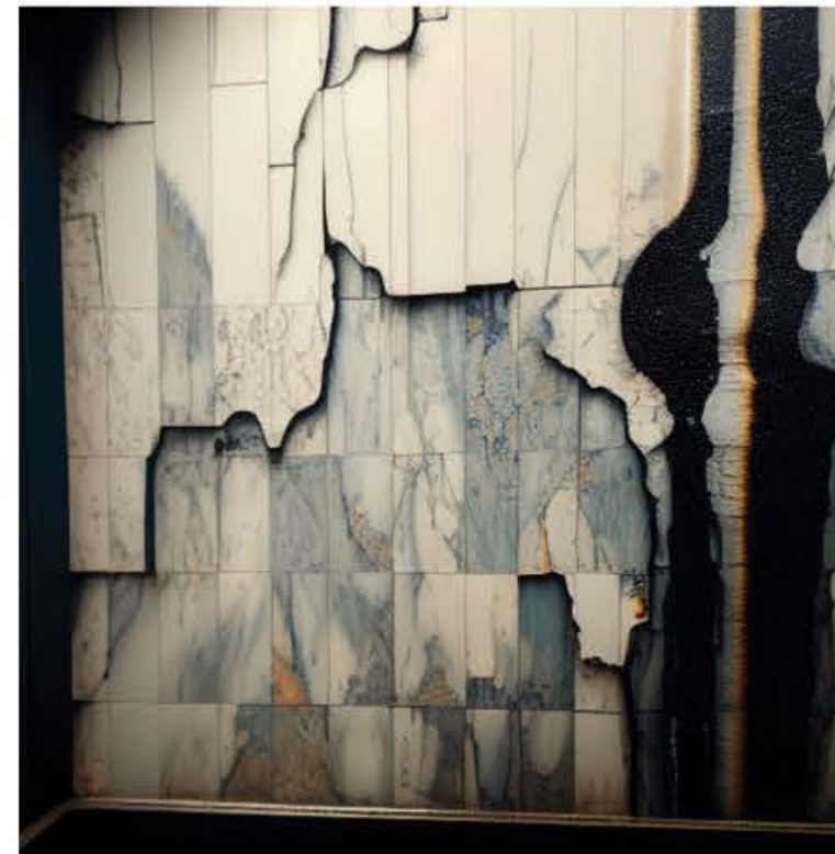
A depressed marble wall
