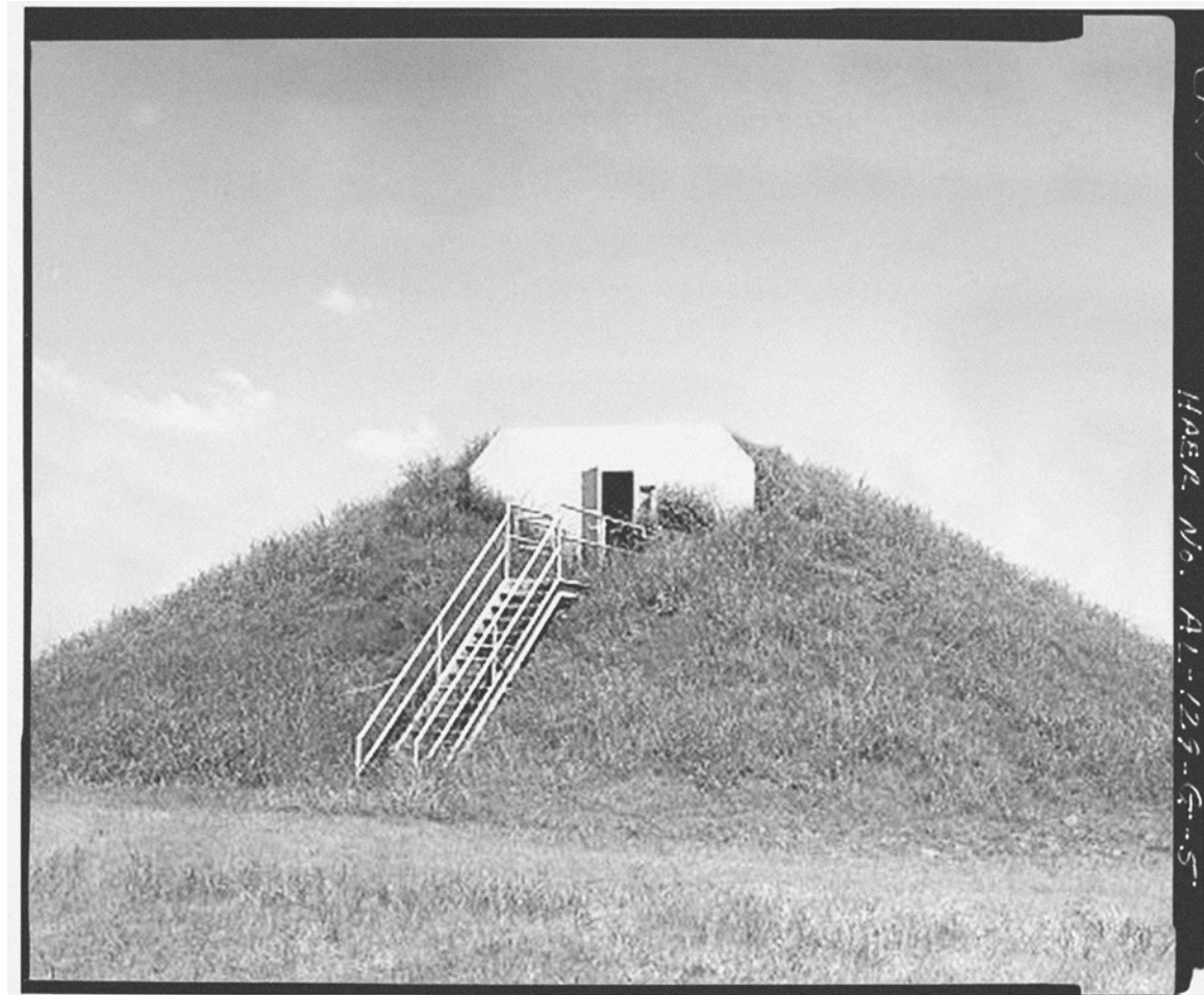
5. VIEW NORTHWEST FROM LEFT TO RIGHT: COLD CALIBRATION OBSERVATION BUNKER BACKGROUND, COLD CALIBRATION TOWER. - Marshall Space Flight Center, East Test Area, Cold Calibration Test Stand, Huntsville, Madison County, AL
