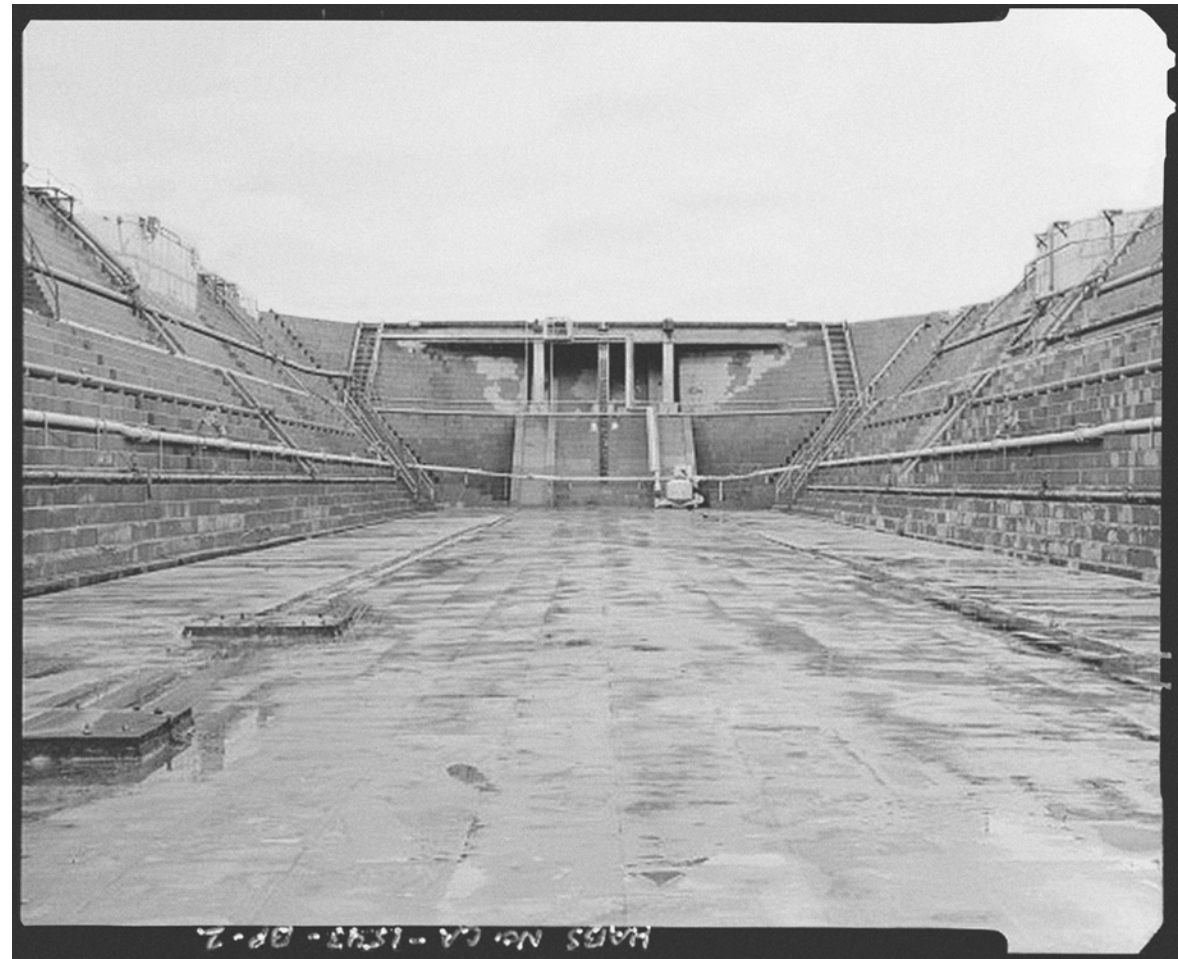
Contextual view of dry dock 1 from west end, showing building 50 and 52 at right; camera facing west. - Mare Island Naval Shipyard, Drydock No. 1, California Avenue, east side near Ninth Street, Vallejo, Solano County, CA
