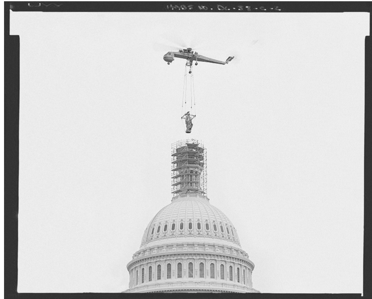
2. View of Statue of Freedom airlifted off of the dome - U.S. Capitol, Statue of Freedom, Intersection of North, South, & East Capitol Streets & Capitol Mall, Washington, District of Columbia, DC
