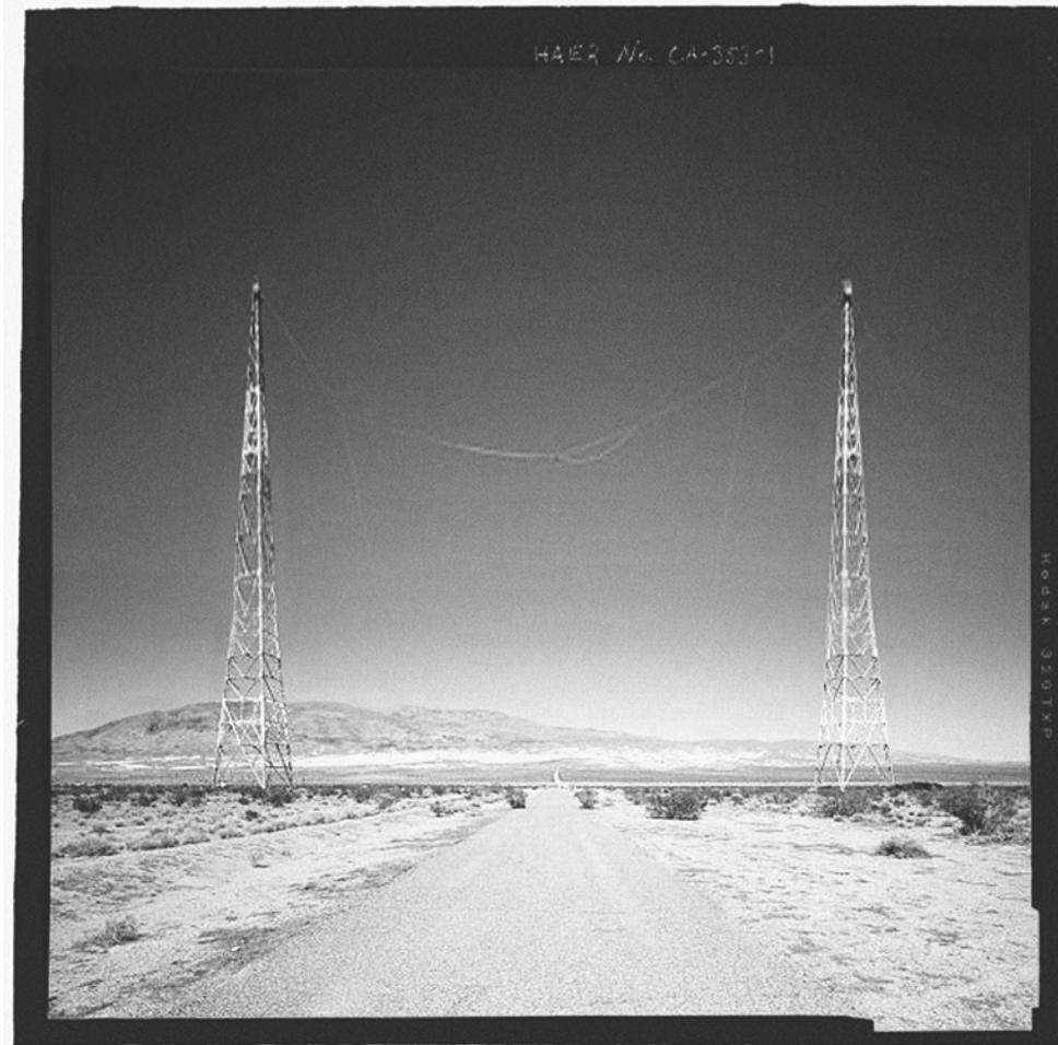
Contextual view of Buildings 70021 and 70022, facing northeast -Naval Ordnance Test Station Inyokern, Randsburg Wash Facility Target Test Towers; Tower Road, China Lake, Kern County, CA
