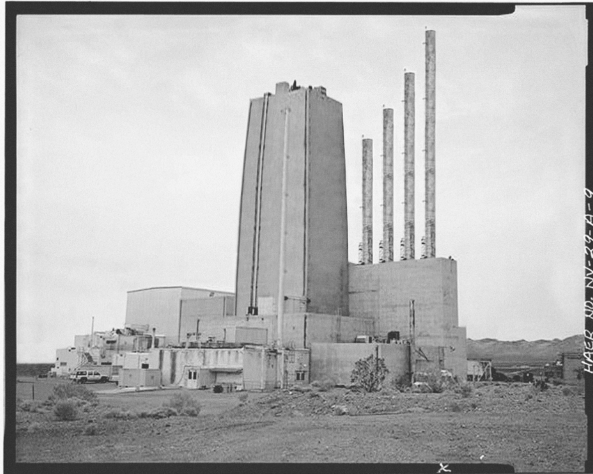
9. EXTERIOR VIEW TO THE NORTHWEST OF THE SOUTH AND EAST ELEVATIONS: - Nevada Test Site, Reactor Maintenance Assembly & Disassembly Facility, Area 25, Jackass Flats, Junction of Roads F & G, Mercury, Nye County, NV
