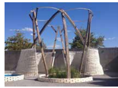
Fig 25 Hy-Fi by the living architects frame detail
