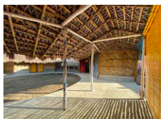
Beyond Survival- Teknaf Upazila, Bangladesh Community Center, Support Facility
